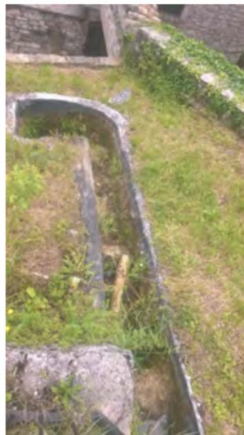
Open channel across the second garden downstream the intake, upstream (left) and downstream (right) ( $B \sim 45$  cm,  $h \sim 40$  cm, drops of the channel bottom  $\sim 30$  cm/1 m).
